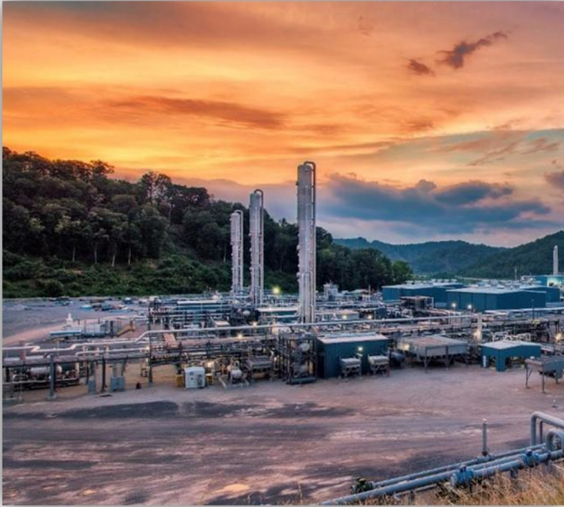
Picture: Sherwood Processing Plant, Marcellus Basin
